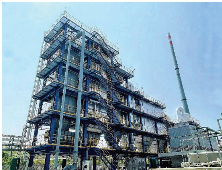
Waste liquid and wastewater incineration system and ancillary flue gas purification device
