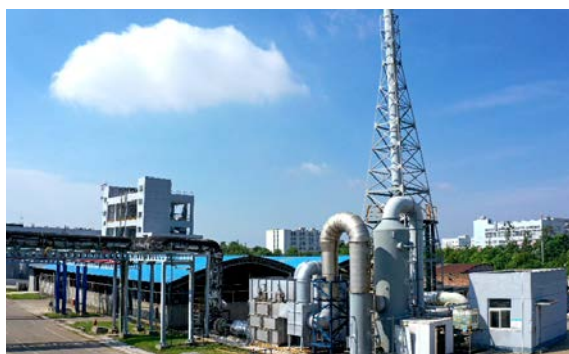
Regenerative thermal oxidizer (RTO) for waste gas treatment
